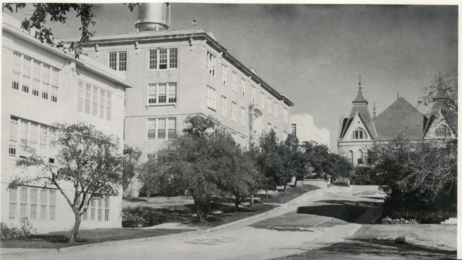
THE HILL is lined with the Education, Science and L. A. buildings. At the top is Old Main.
